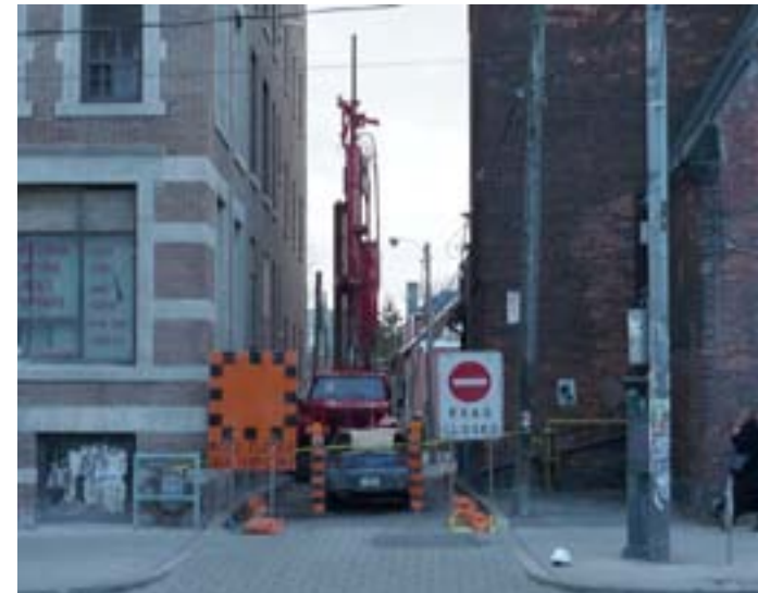
Figure 2 - Drilling in the public laneway at Planet Traveller
